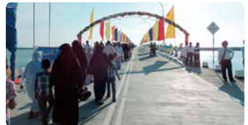
Manmunai Bridge, which was completed in April 2014 (Sri Lanka)
