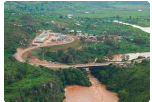
The OSBP Facility and Rusumo International Bridge (at the border between Tanzania and Rwanda)
